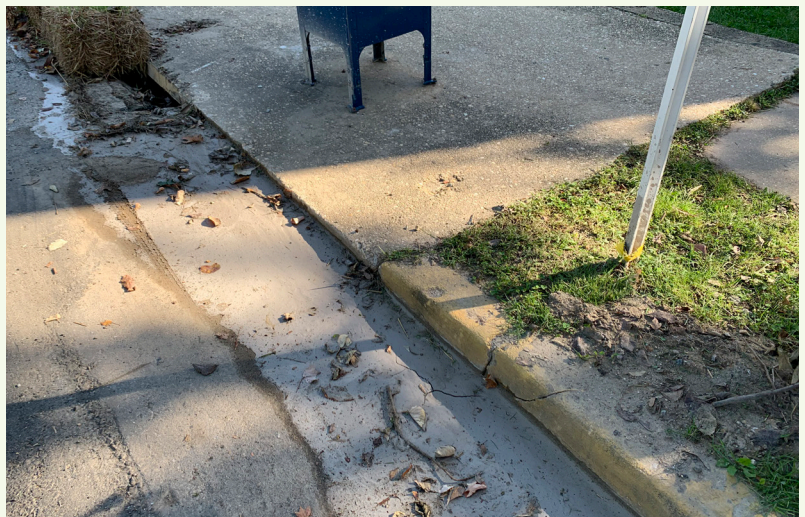
Sediment from upstream construction site entering storm drain inlet.
