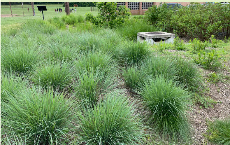
Ornamental grasses provide stabilization on the BMP side slopes
