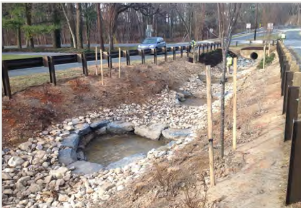
A step pool storm conveyance system (SPSC) during the installation process (left), and post-construction (right). While not detailed in this guidebook, SPSCs can provide slope and outfall stabilization.
