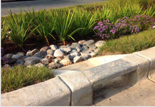
Close-up of a stormwater inlet along Dennis Avenue
