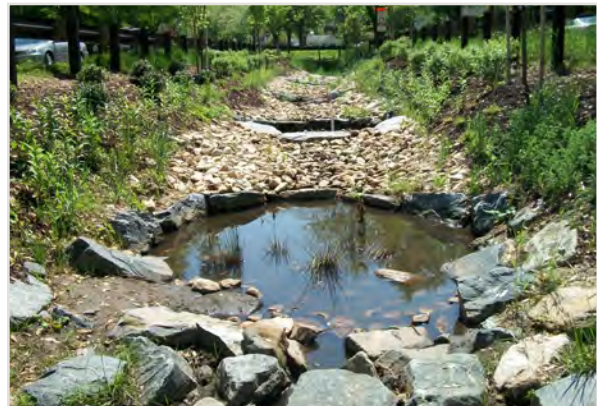
A step pool storm conveyance system (SPSC) during the installation process (left), and post-construction (right). While not detailed in this guidebook, SPSCs can provide slope and outfall stabilization.
