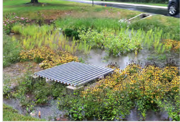
An overflow riser installed along Dennis Avenue
