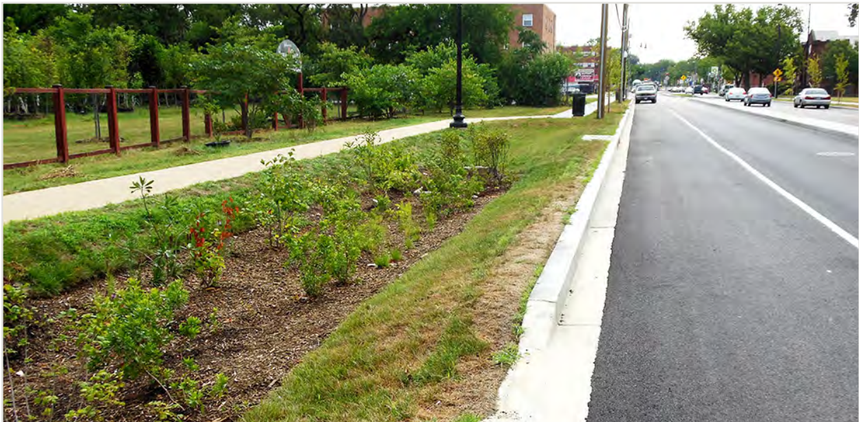
A bioswale is added along the street.
