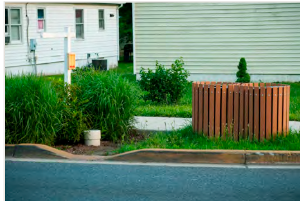
Stormwater curb extensions installed along Decatur Street (top and middle). A close-up of a stormwater outlet (bottom).
