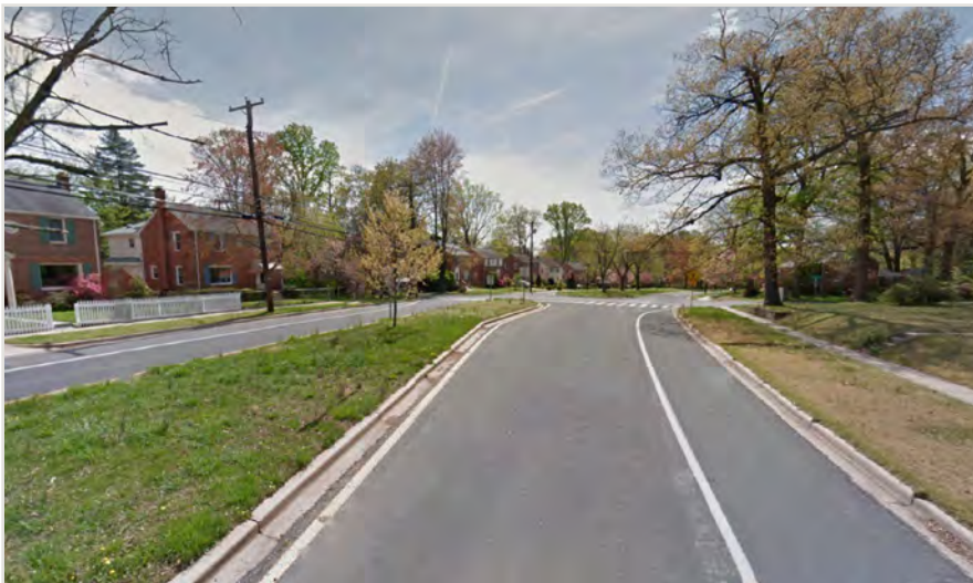
FIGURE 4.10. EXAMPLE OF A TYPICAL MEDIUM-DENSITY RESIDENTIAL STREET
