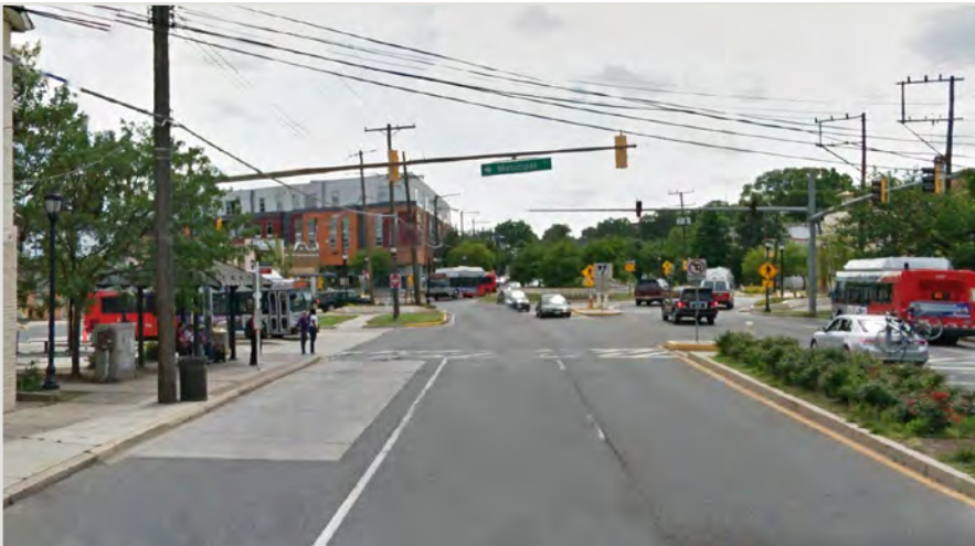
FIGURE 4.1. EXAMPLE OF A TYPICAL DOWNTOWN COMMERCIAL STREET
