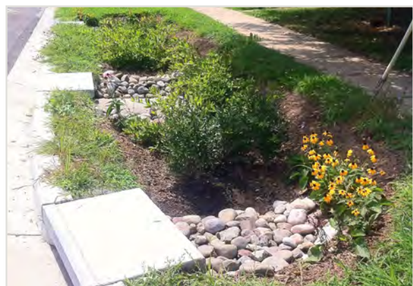
A bioswale after construction
