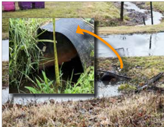
Figure 25. Existing culvert under 41st Street trail. Areas is near Northwest Branch trail intersection.
