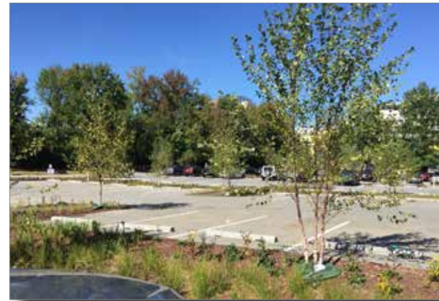
Figure 40. First United Methodist Church (after). The lot was redesigned to incorporate permeable parking pads and bioretention.
