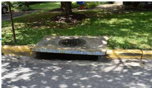
Figure 15. Existing storm drain inlet along 41st Place
