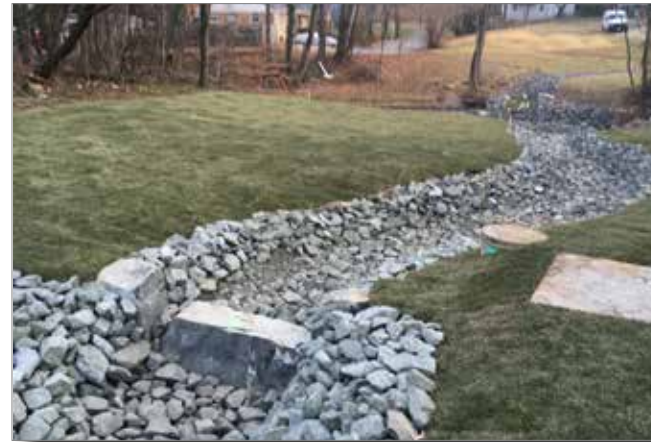
Figure 18. Outfall stabilization project in Suitland, MD
