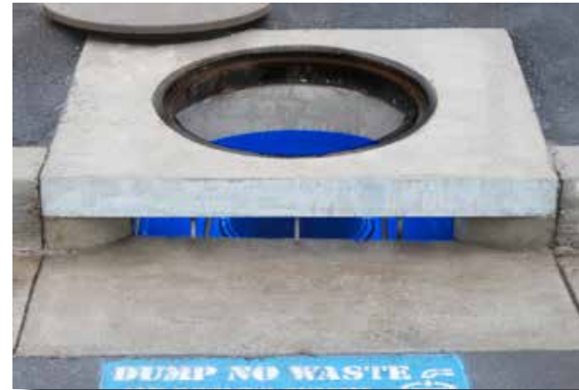
Figure 16. Example of a curb inlet storm drain insert
