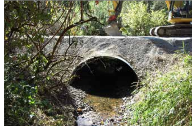
Figure 26: Culvert replacement project under a park trail
