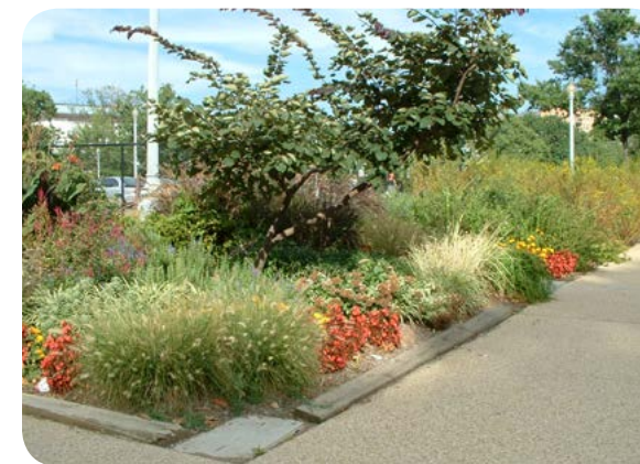
Bioretention basins (rain gardens) allow rain and snowmelt to seep naturally into the ground while also providing beauty in the landscape.
