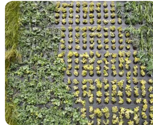
A plug system can be used in an interior setting combined with rainwater harvesting and filtering system.
