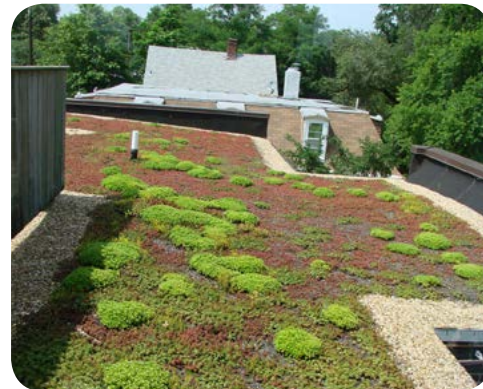
Research conducted on green roof installations in the Midwest indicates that they can retain an average of 75% of annual rainfall, with winter absorption averaging 40-50% (MacDonagh 2005).
