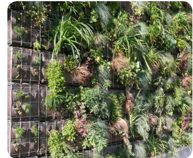
A tray system is where soil is bound in burlap and plants are inserted through a hole in the fabric.
