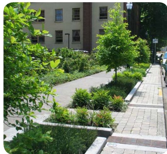
Stormwater planters are an on-site retrofit option for treating rooftop runoff in ultra-urban areas.
