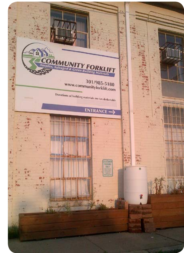
A rain barrel installed at Community Forklift in Edmonston, MD.
